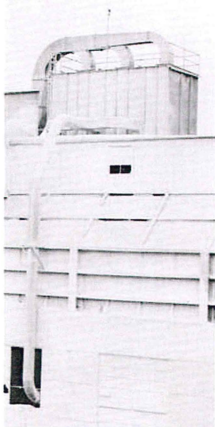
(Above) The Wheelabrator Dustube Collector is located on top of building where railroad cars and trucks are loading.
